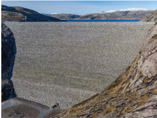
Svartevatn Dam (Photo: Sira Kvina)
