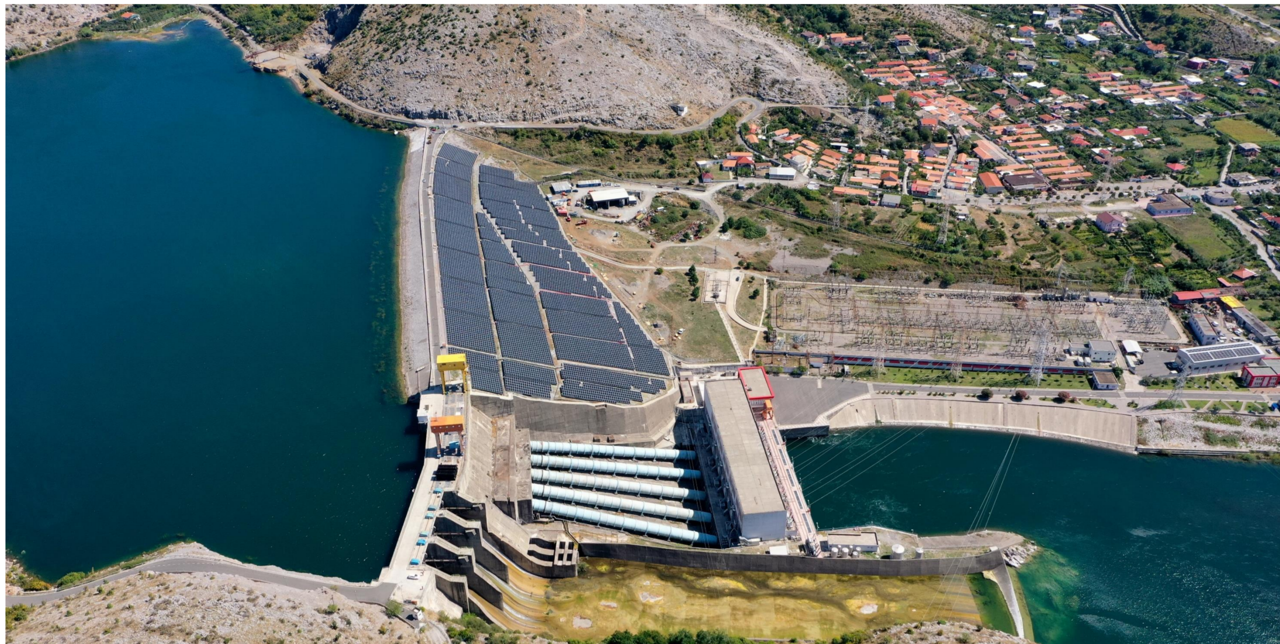
Figure 1: View of PV Plant on the downstream face of Qyrsaq Dam
