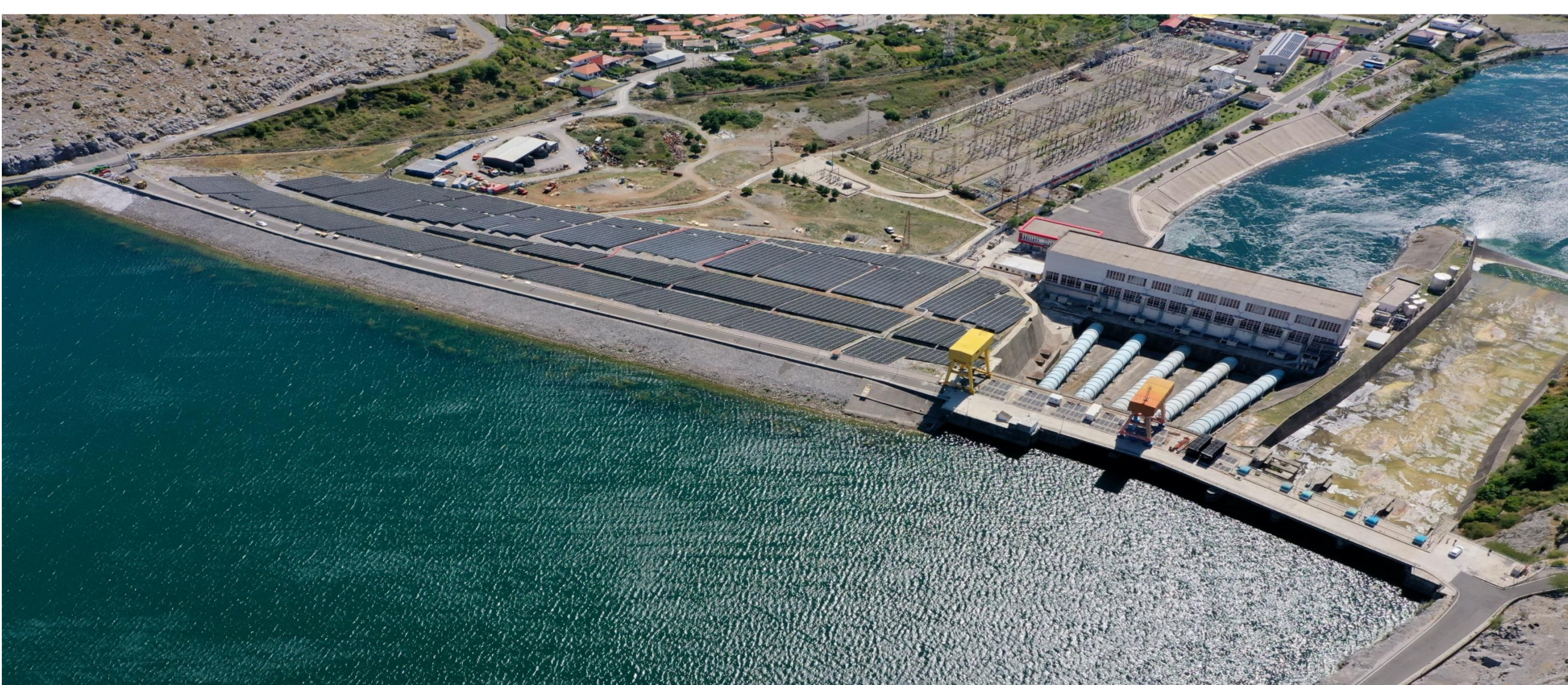
Figure 2: View of PV Plant in Qyrsaq Dam from Upstream
