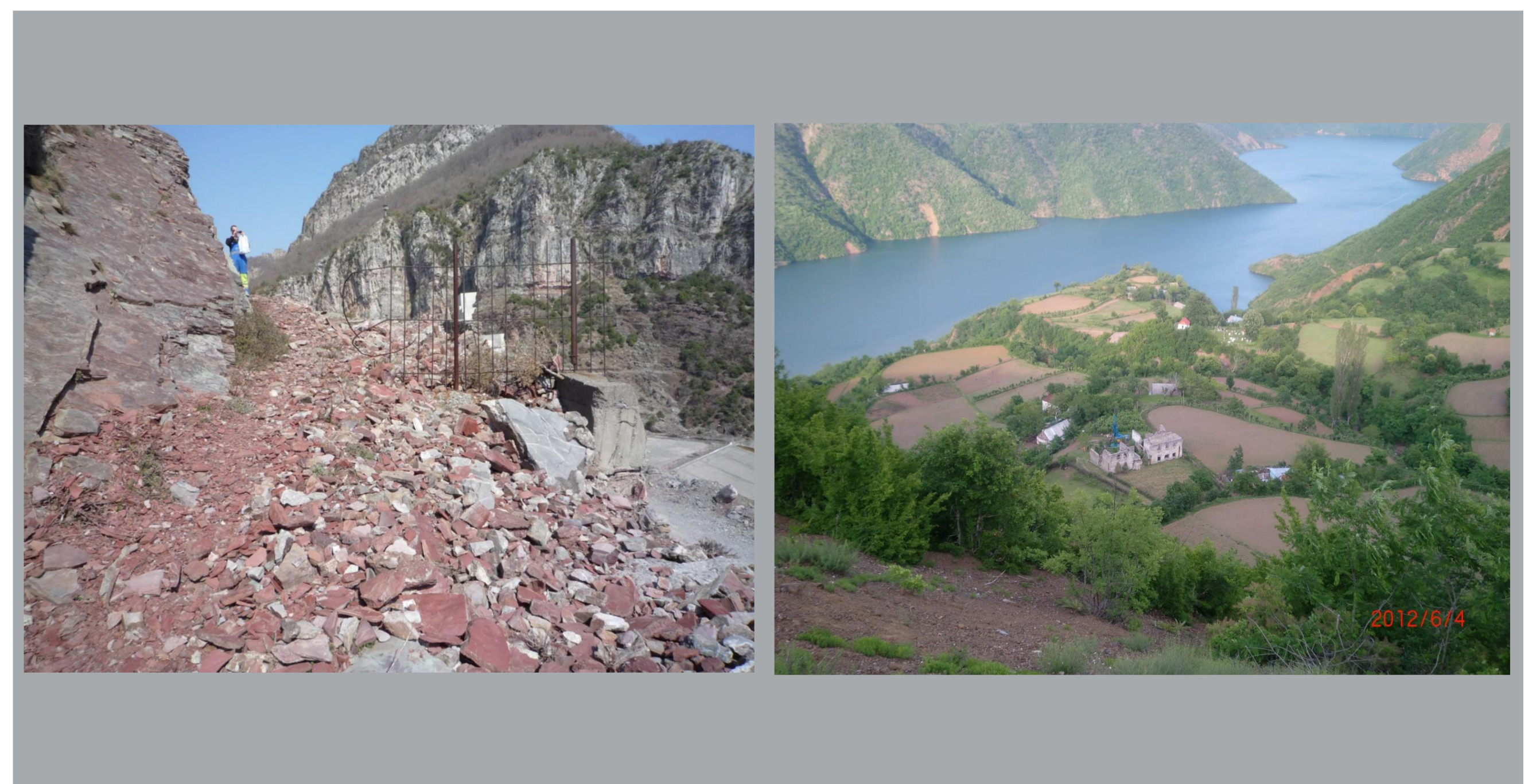
Fig. 3: Geohazards present at Komani and Fierza dams' area
