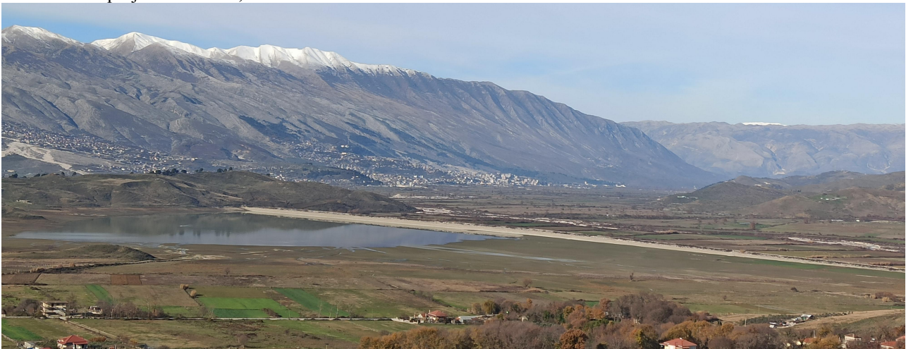
12- Irrigation dam and reservoir of Stropcke, Pogradec, H = 40.0 m, Reservoir projected volume, Vu= 1.5 milion m3
