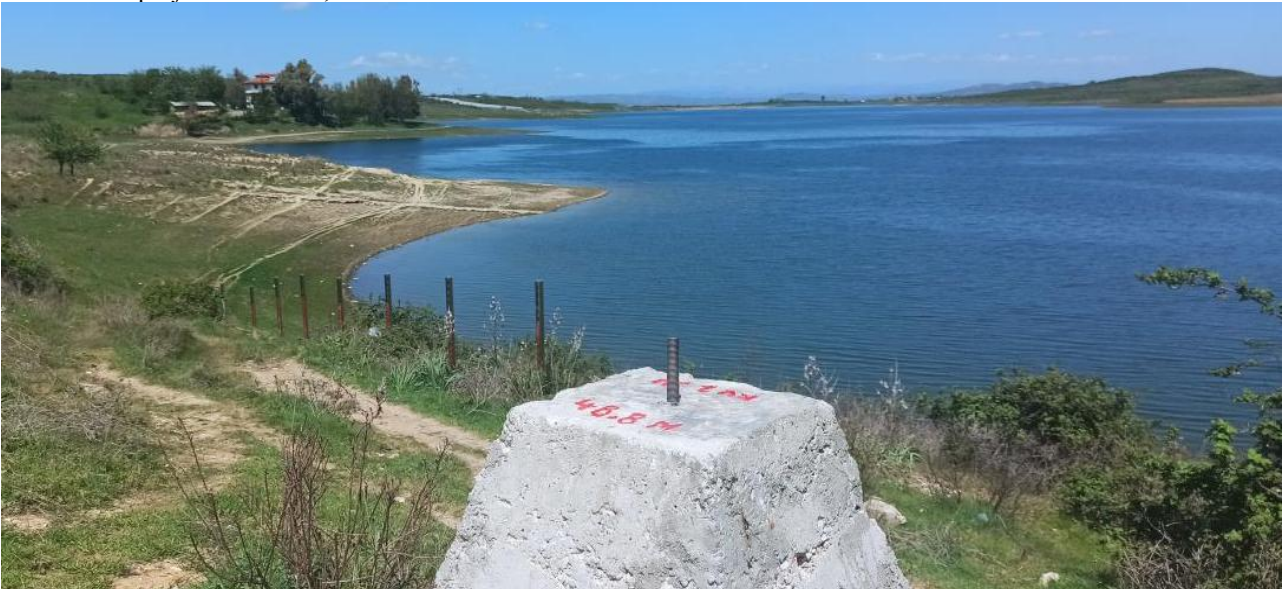
9- Irrigation dam and reservoir of Murriz Thane, Lushnje, H= 12.46 m, Reservoir projected volume, V_u= 60.0 milion m 3
