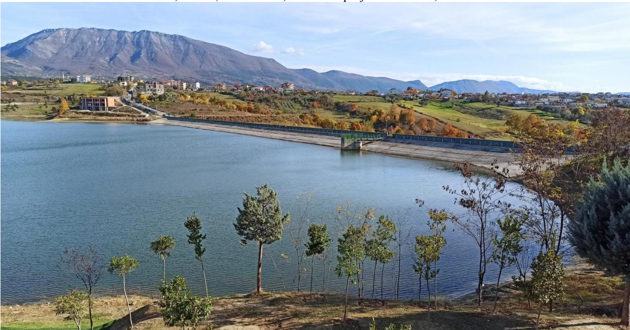
6- Irrigation dam and reservoir of Koshnica, Devoll, H = 31.0 m, Reservoir projected volume, Vu= 3.7 milion m3
