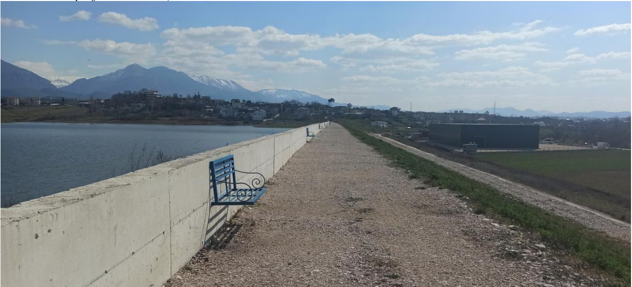
14- Dam and Reservoir of Paskuqan, Kamze, H=28.0 m, Reservoir projected volume, Vu=9.0 milion m3
