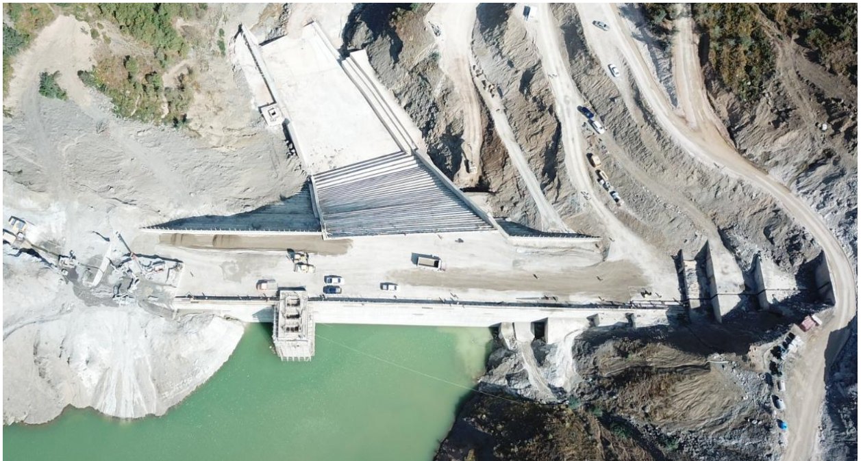
Overview during the construction, 2018
