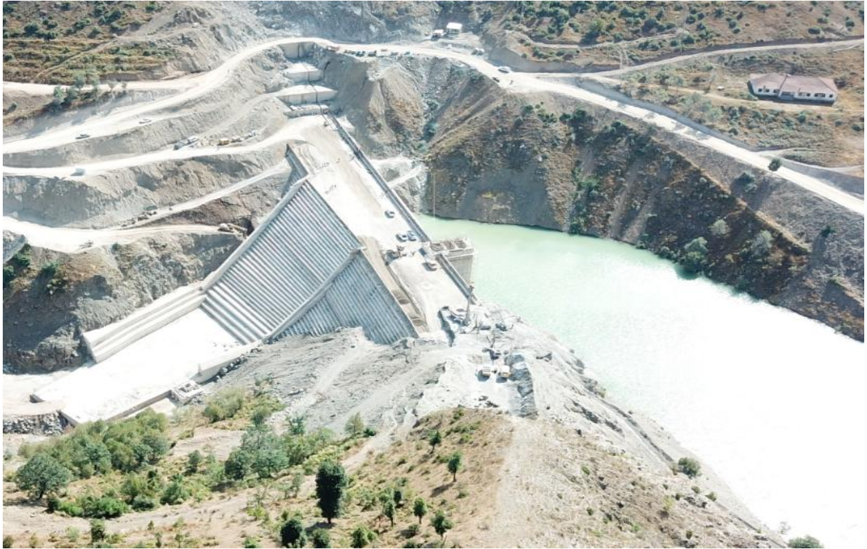
Overview during the construction, 2018
