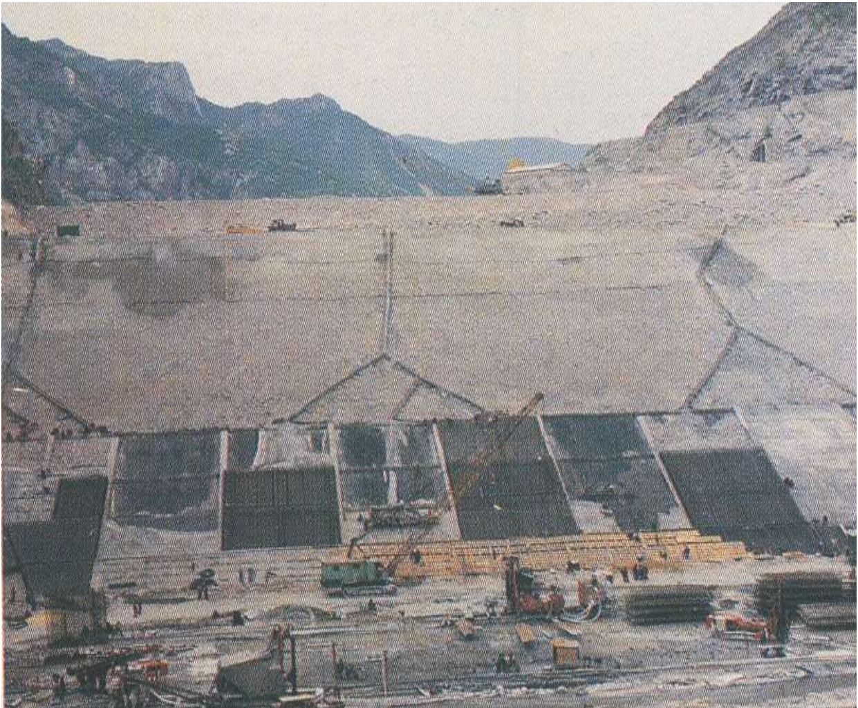
During construction of reinforced Concrete Face of Dam, HEPP Koman
