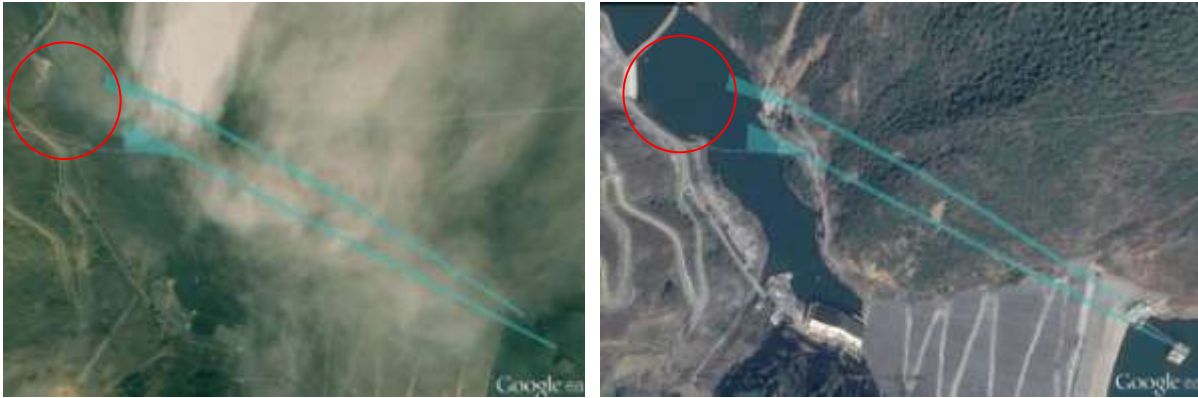
Figure 2: Jets' alignments (cyan) on satellite images. 2003 with three span bridge (left); 2013 with eroded left bank and two additional bridge spans
