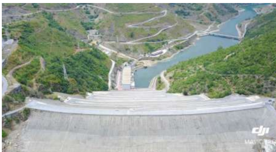
Figure 1: Fierza Dam. View of downstream zone from the crest
