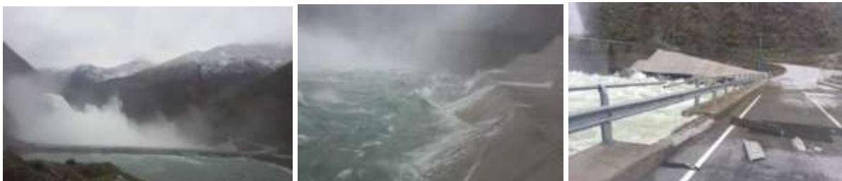
Figure 4: View of Discharges of 600 \text{ m}^3/\text{s} from Spillway No. 4, November 2016 and Waves on the left bank protection (left) and associated damages associated to Spillway No. 4 in operation at 50%
