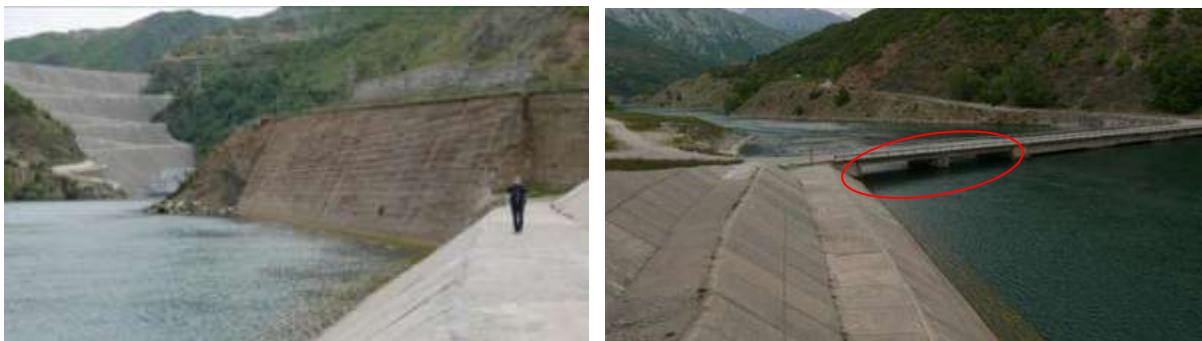
Figure 3: Left bank protected area (left) and two new bridge spans (right)
